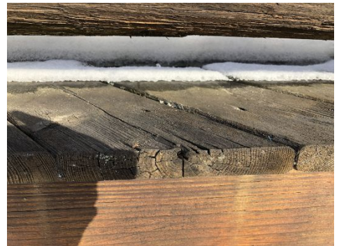
Limited view of deck boards due to snow, but some were rotting.
