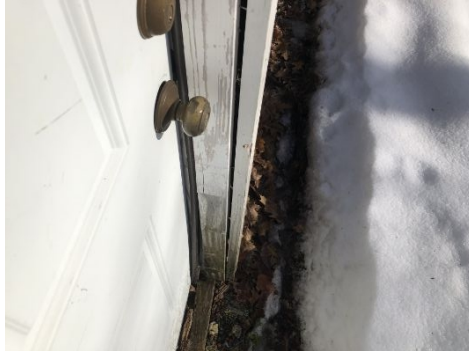
Door under porch area was damaged and installed incorrectly. Weathered and damage observed
