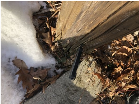
Missing joist hangers
