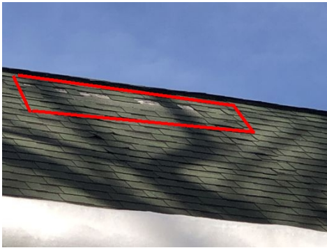
Missing shingles, exposed sheathing
