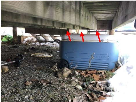
Missing joist hangers
