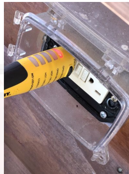
Outlet in porch area appeared to have an open neutral and was not working.
