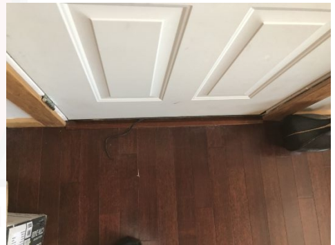
Door onto the porch had damaged weatherstripping
