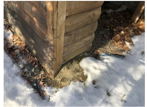
Log siding was below ground level, wood rot was observed
