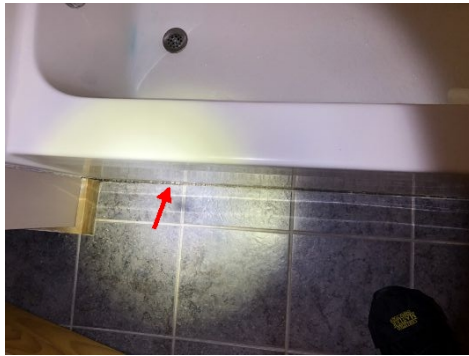
Both tubs need to be sealed where it meets the floor, large gap observed
