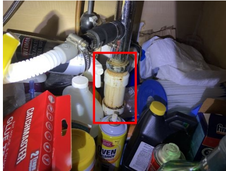
Under kitchen sink, past signs of staining
