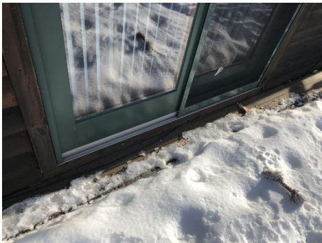
Sliding door was difficult to slide open and close. May need to be adjusted or lubricated.
