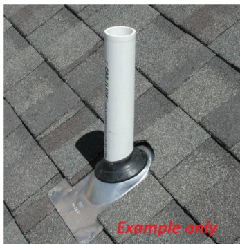
Sample of proper installation
