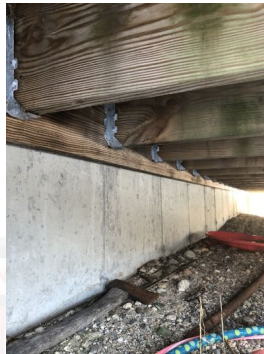
Missing lag bolts from ledger board
